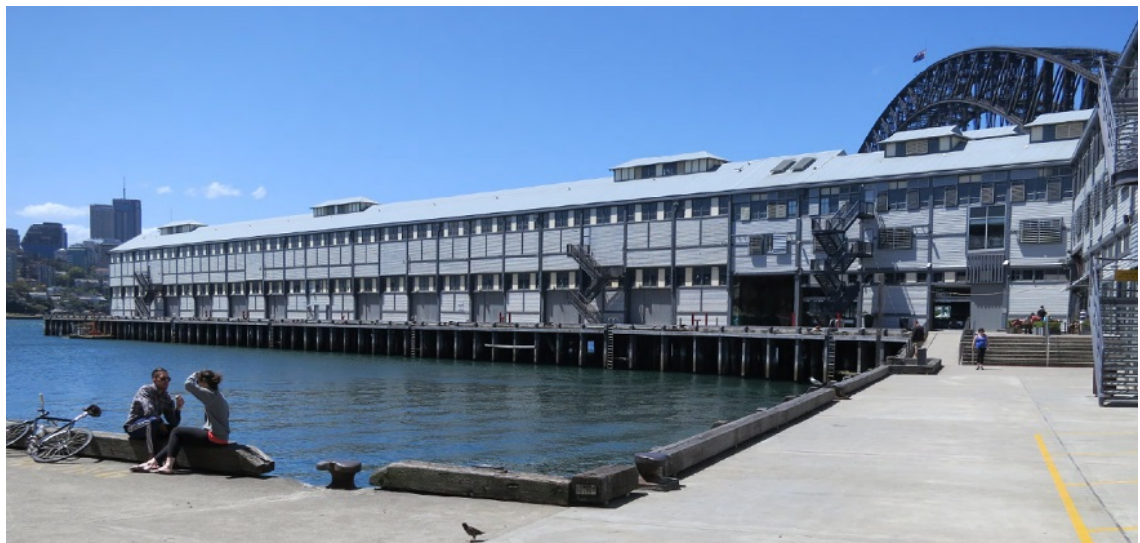
Figure 3: Pier 2/3 looking north
